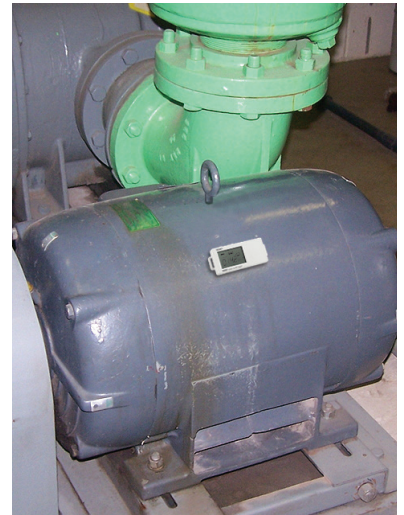
HOBO UX90-004 Motor On/Off data logger records motor on/off status.
