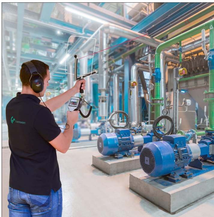
Accurate leak detection during operation with laser pointer and integrated camera
