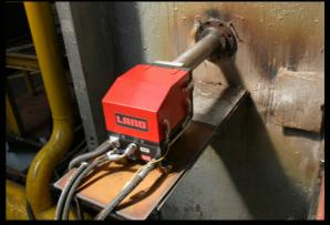
Typical installation showing the FTI-Eb mounted into a process - the sensor is shown in the protective ensclosure
